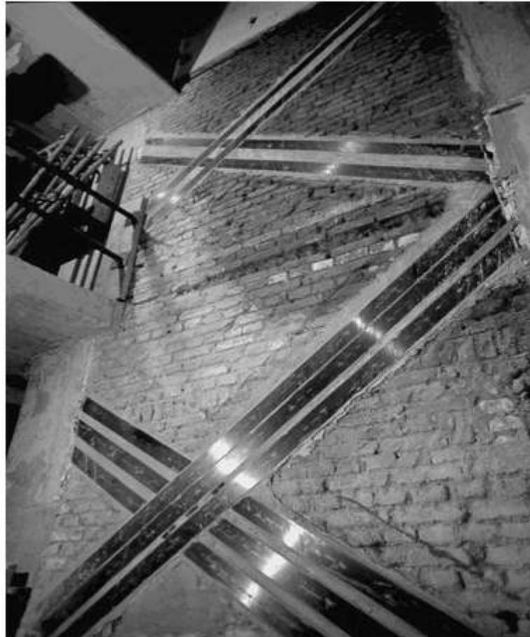
13.11 Strengthening masonry wall (photograph by courtesy of Sika Ltd).
